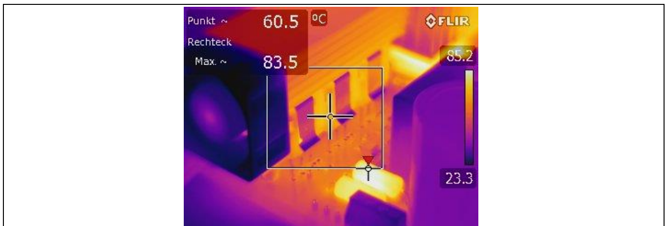
Figure 34 Thermal image of evaluation board at 18 kHz switching frequency, 10 Ω gate resistance and forced convection
